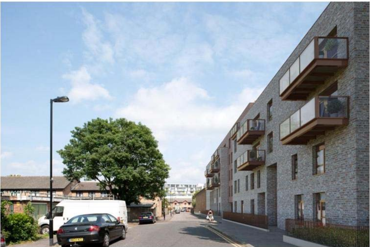
View looking east along Miles Road
