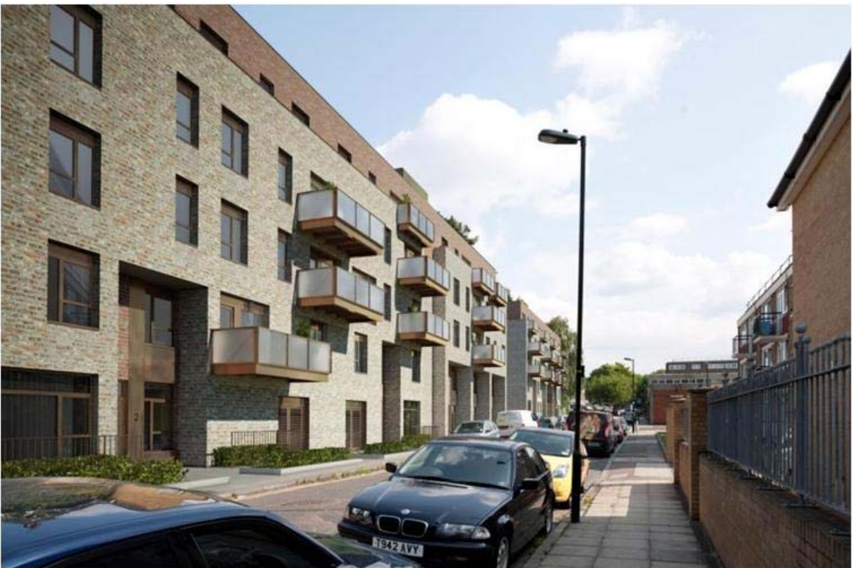
View looking south along Myddelton Road
