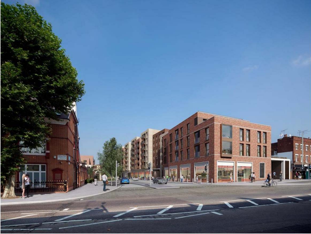
View from High Street
